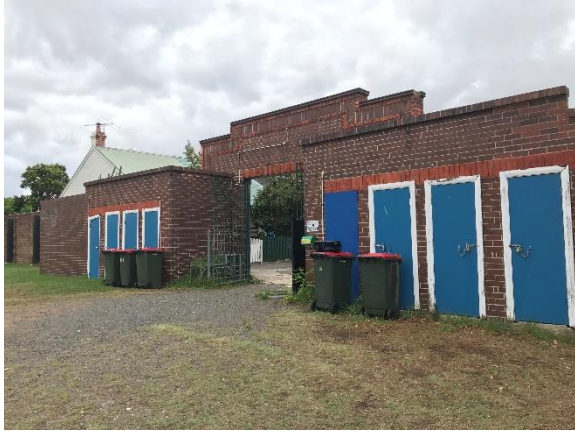
Photo 1. No access to interior of the building at the time of assessment. No hazardous building materials suspected at the time of assessment.
